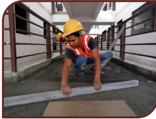
Floor Tiling work training
