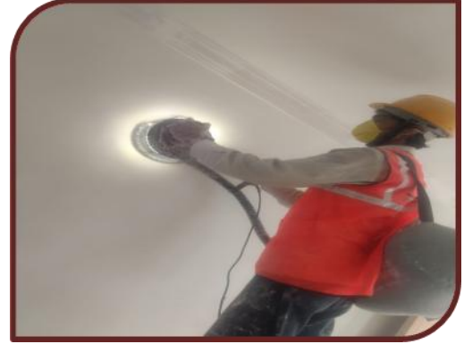
Wall leveling work at site
