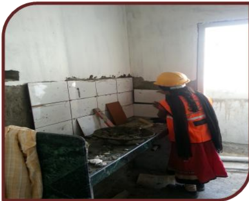
Women doing Tiling work at construction site
